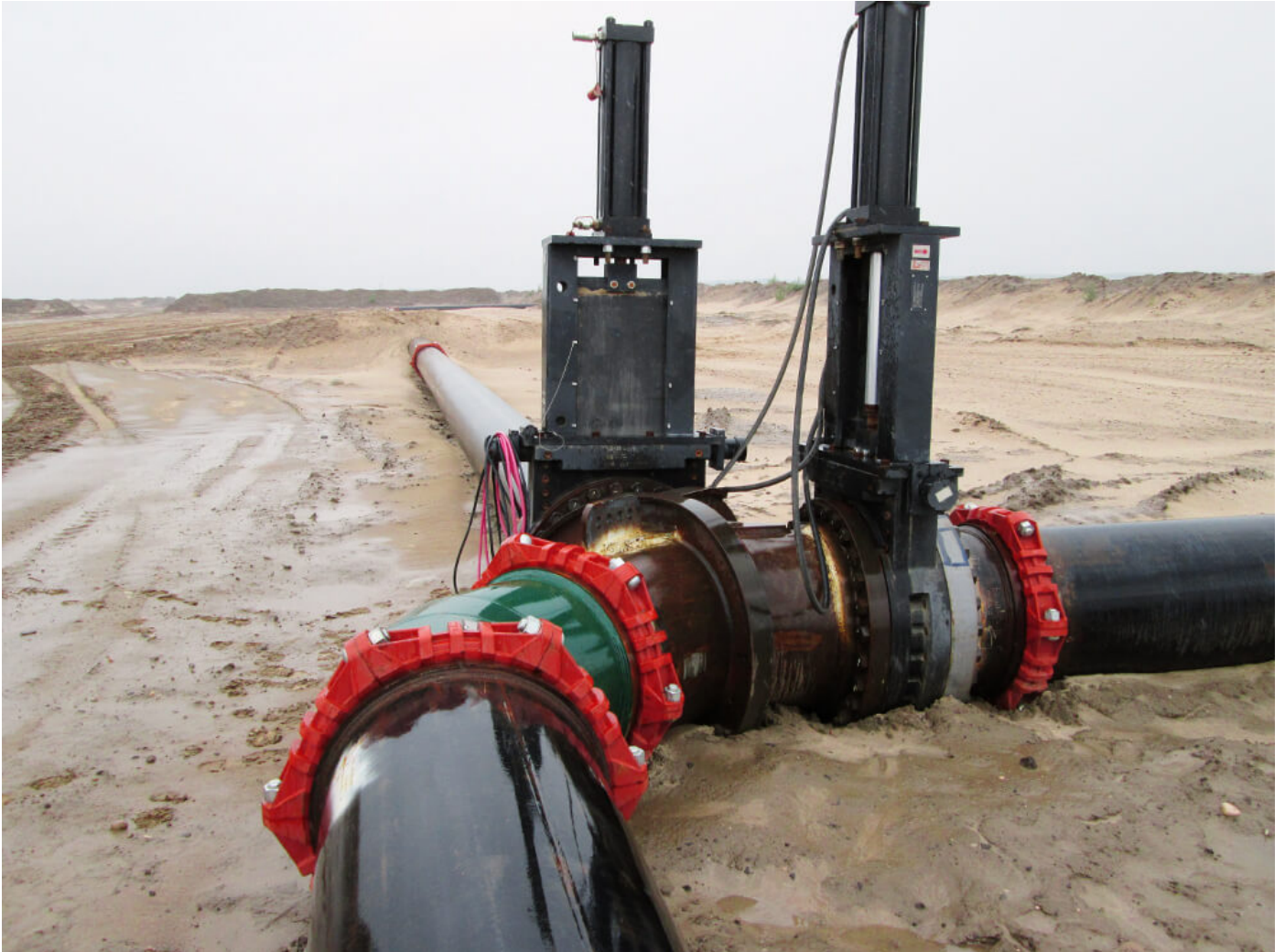
Wey W3 with hydraulic cylinder in an oil sands mine in Canada.
